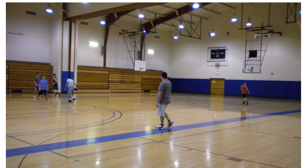
The existing Dods gym does not have sufficient capacity for basketball and volleyball competition requiring games to be played on the rubber floor of the Steele Field House.
