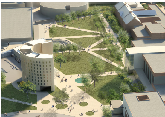
Main Quad Renovation
