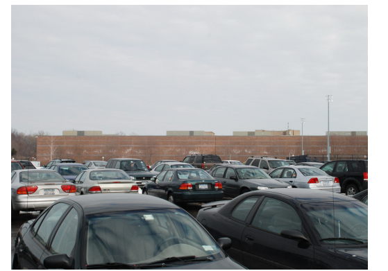
15. View from Ring Road over the parking lot towards Steele Hall. The long windowless façade creates a severe edge in winter, when the deciduous trees in front of have lost their foliage.
