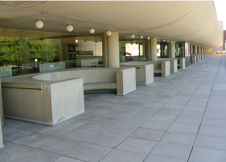
Sculpted concrete sitting niche at the Library Plaza.
