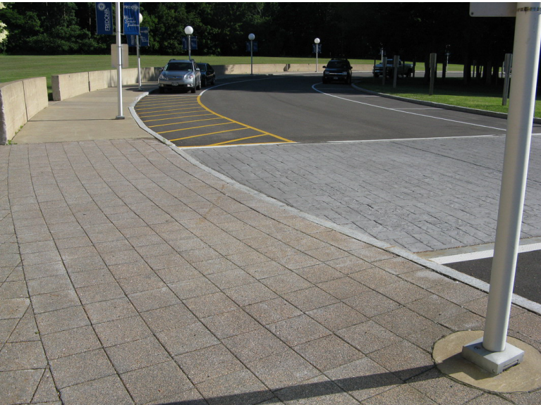
Range of site materials: buff-colored concrete sidewalks and walls, concrete pavers, stamped concrete crosswalks.
