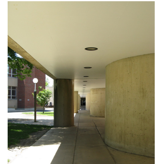
The Spine lower passageway is one of the major pedestrian routes.
