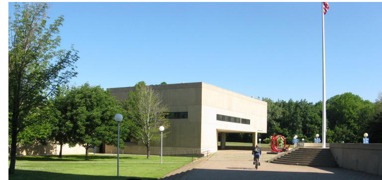
Bicycle racks are provided near most building entrances.
