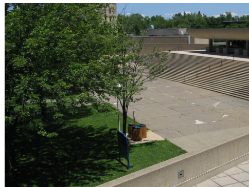
Library steps and Plaza as seen from the Spine. The vast plaza paving is in need of repair or redesign.
