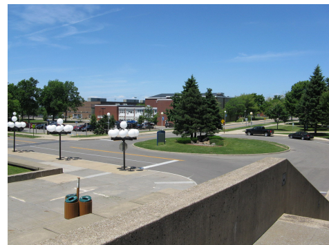
3d. The traffic turnaround as seen from the Spine. Ring Road is to the left.
